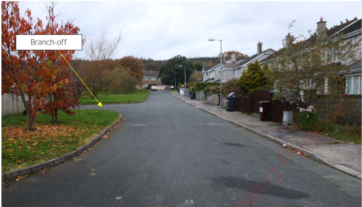
Figure 2-19: Site access road (Looking North-West)
