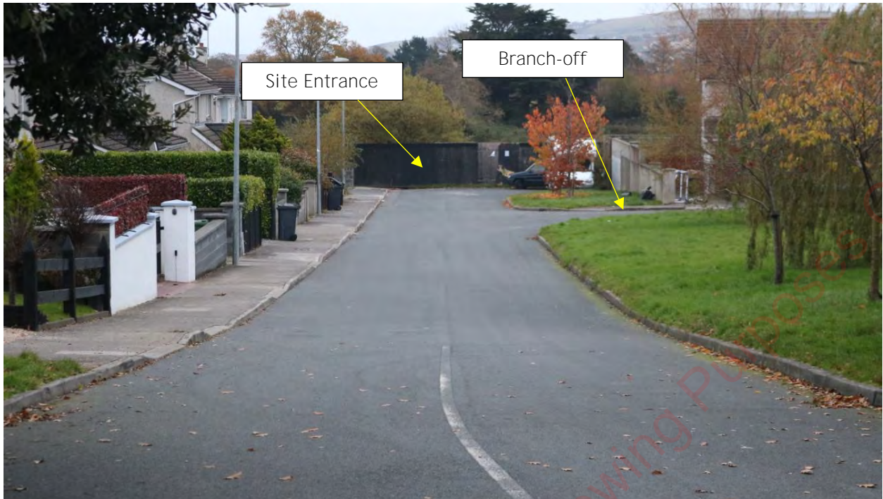
Figure 2-17: Site access road looking towards the site entrance (Looking South-East)
