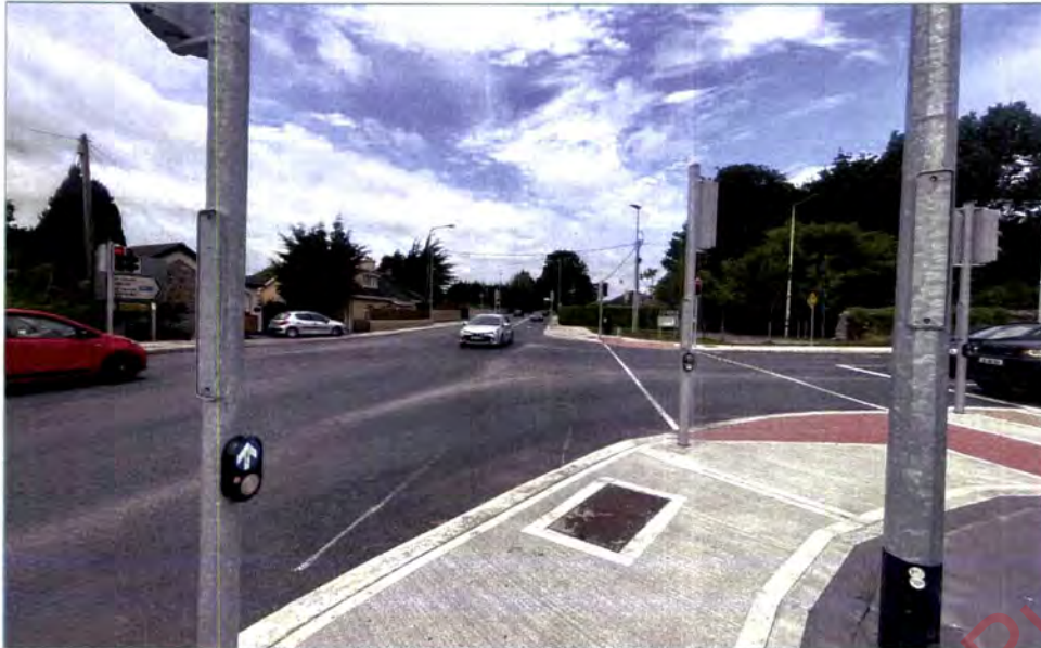
Figure 2.5 – R722 / R761 Signalised Junction
