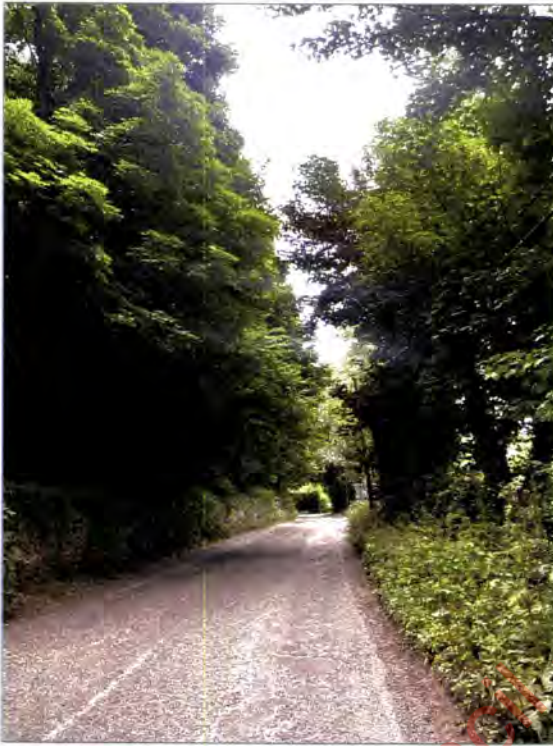
Figure 2.4 – R761 North South View
