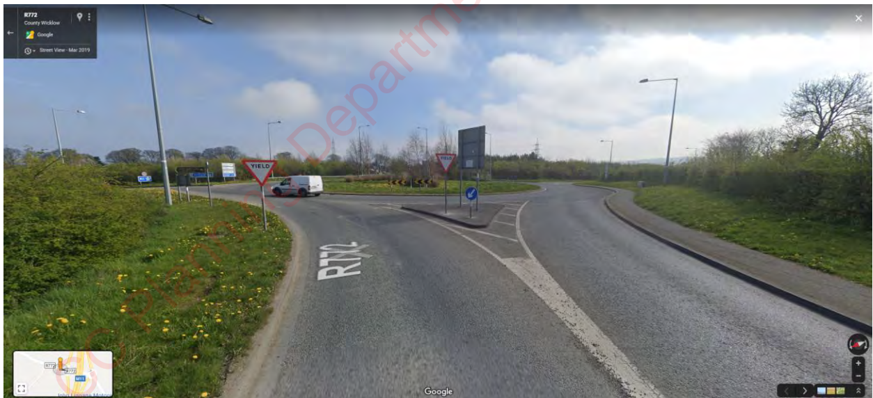
Figure 2-4: R772 Roundabout junction with M11 Junction 16 (Looking South East) © Google Maps
