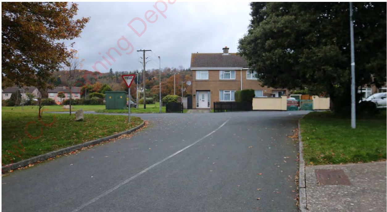
Figure 2-16: Site access road (Site 4) (Looking North-West)
