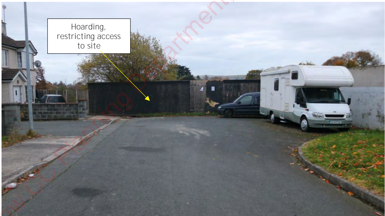
Figure 2-20: Site Entrance (Looking South-East)
